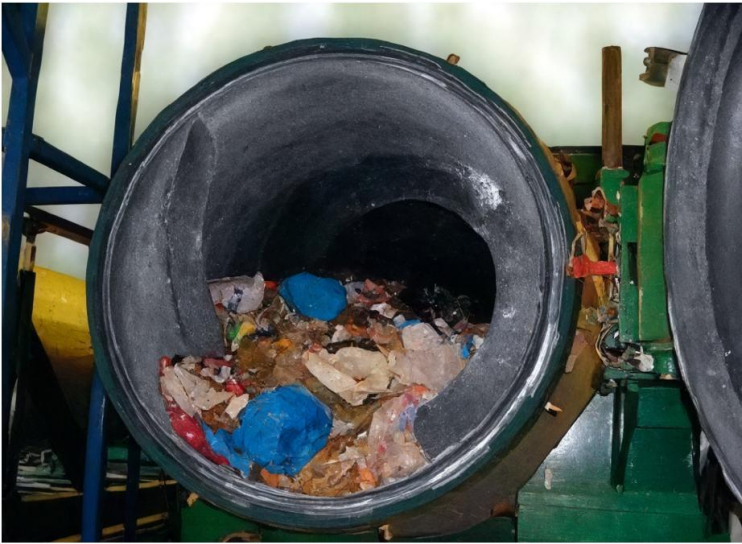
FIGURE 6: Detail of MSW feeding in autoclave.
